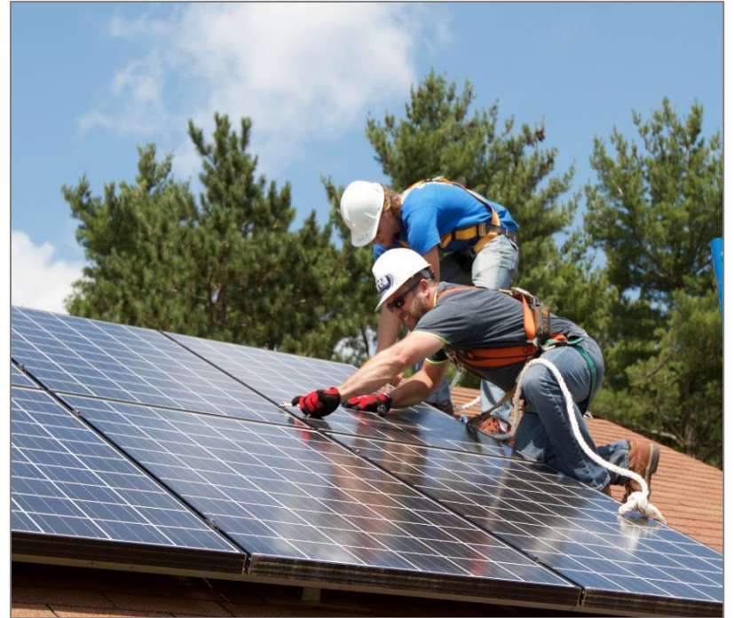
Students configuring a roof-mounted system on MREA's training roof.
